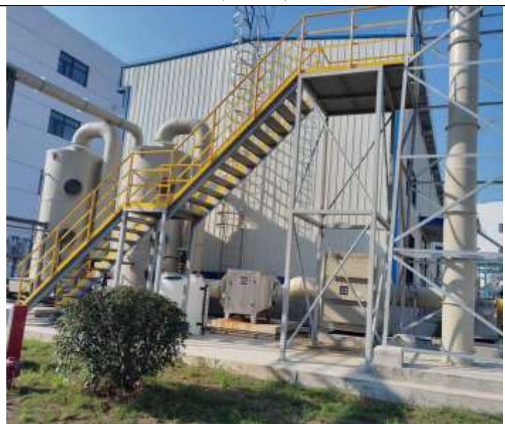
一级碱喷淋+一级水喷淋+干燥+两级活性炭吸附-脱附 (TA003)
