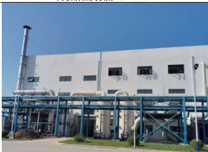
一级碱喷淋+一级水喷淋+干燥+两级活性炭吸附-脱附 (TA002)
